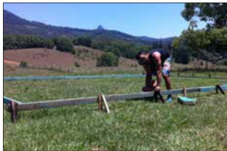
Sridas starts the formwork on the Hanuman House project.
